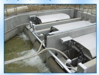
☐ The cleaning and rinsing of filter cloth is maintained automatically during filter operation. Clear, already filtered water is used for rinsing; hence there is no need to couple on a process water unit.
