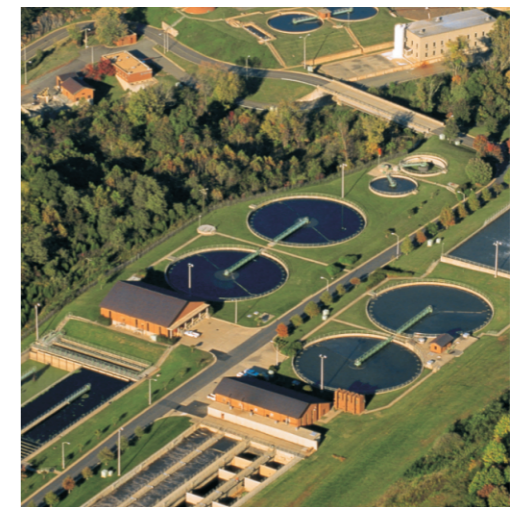
~Waste water treatment in industry
