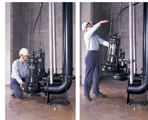
~Tos-Guide Rail System Installation
