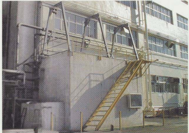
General view of facility
